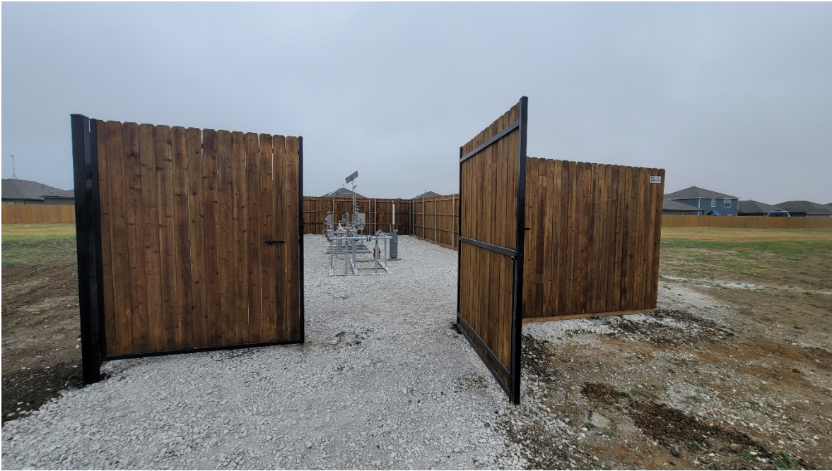
Figure 3: Crushed Gravel & Swing Gate
