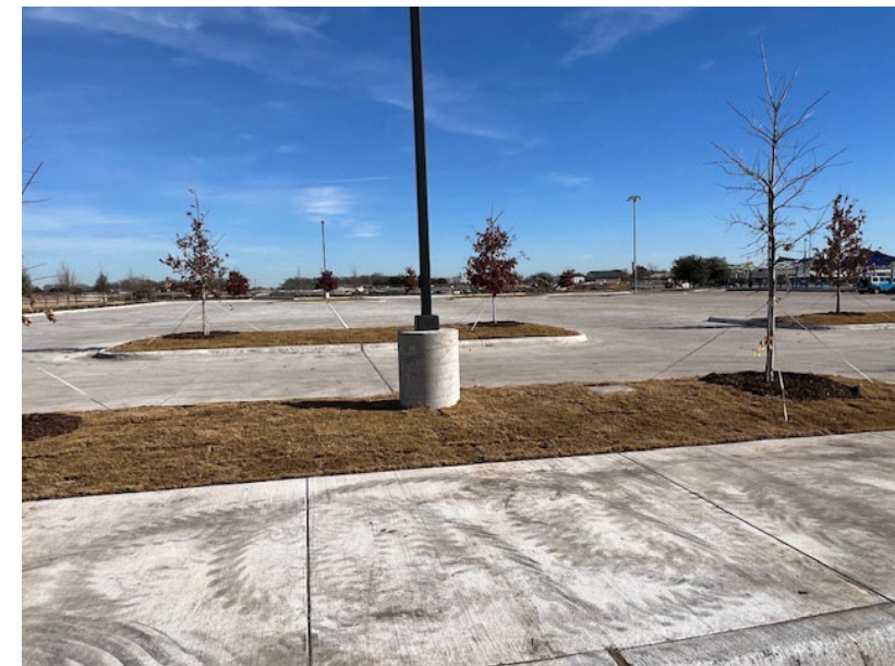
DECEMBER – Parking Lot
