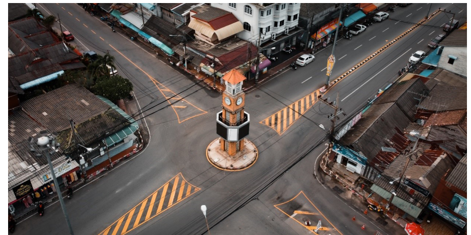
Exhibit 6.15: Roundabout Example Photos
